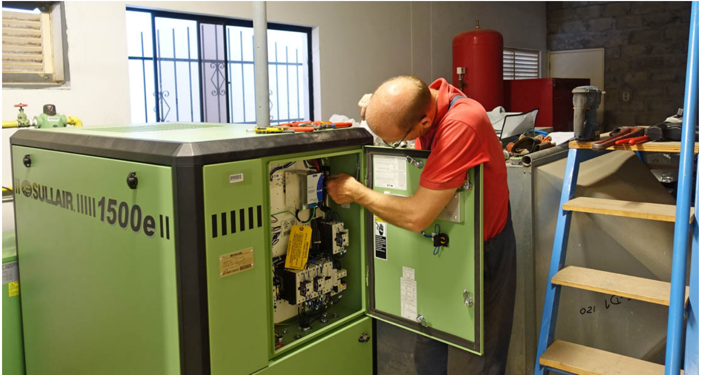
Connecting the new compressor.
