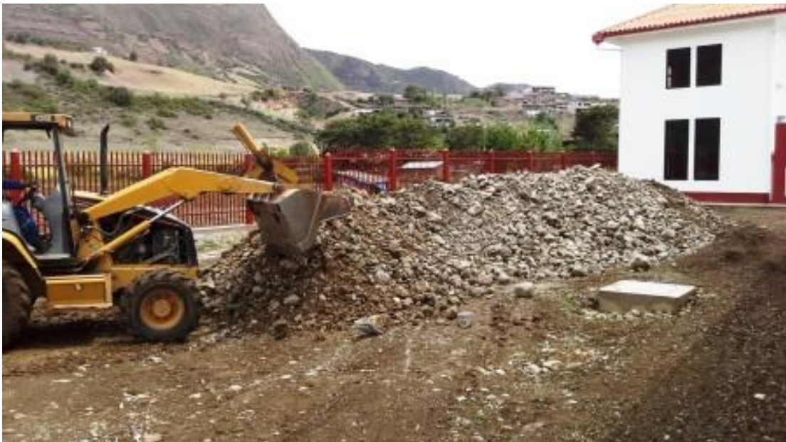
Moving dirt for the school garden.
